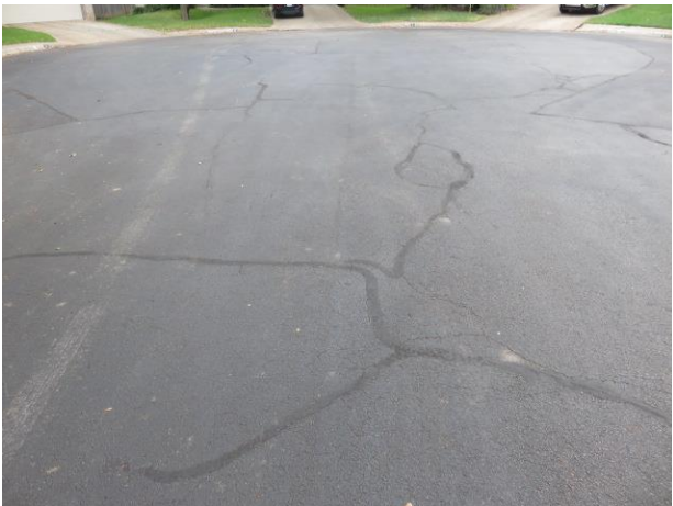
Crack repairs at cul-de-sac
