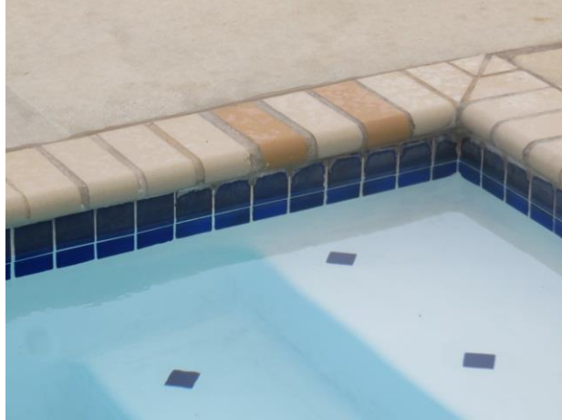
Partial coping repair
