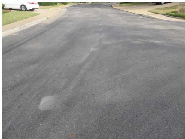
Side street pavement in good condition
