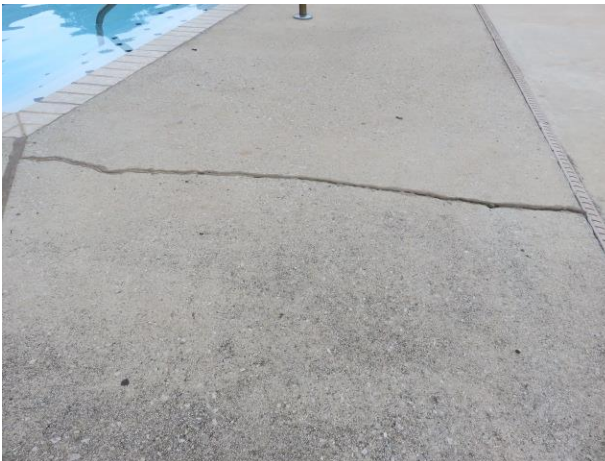
Repaired crack and settlement
