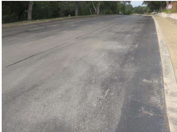
Repaired longitudinal cracks at centerline and edge
