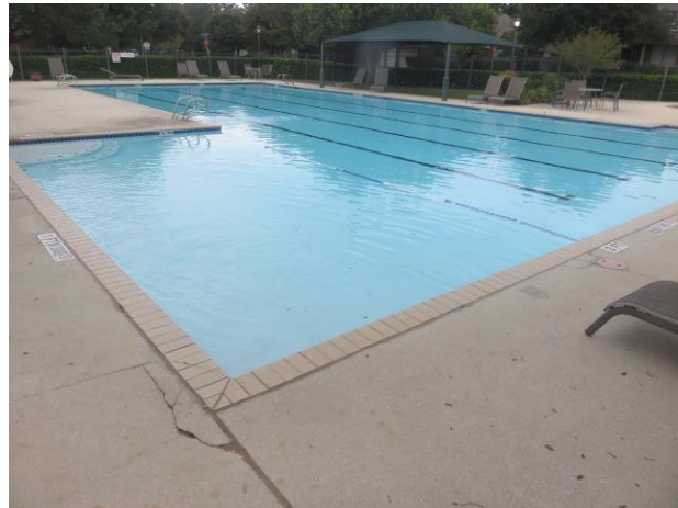
Pool structure with plaster pool finish
